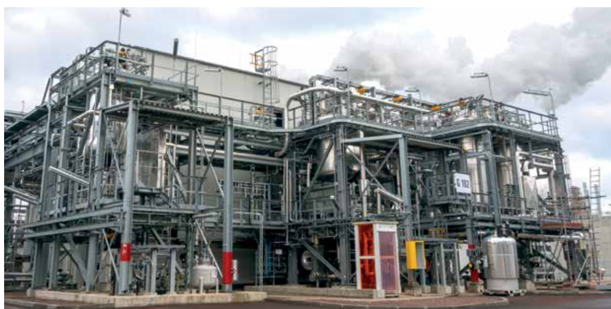
S-SBR pilot plant for the production of new rubber materials for high-performance tires
