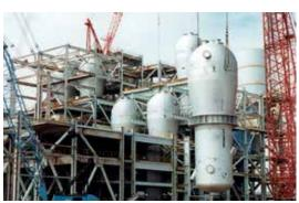
tors, containers, production assembly and piping are fixed on a steel framework, which is 100 m high. Pörner was charged with calculations for 16 reactors according to Australian standards, 17 different apparatus and about 20 piping systems.
