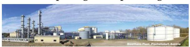
PISCHELSDORF. **AGRANA** Bioethanol GmbH put up the largest Bioethanol plant in Austria. There alcohol is produced out of agricultural commodities, and afterwards blended into petrol. As general planning contractor Pörner was commissioned with all related engineering scopes, like construction engineering, static, steel construction, processing plant equipment, piping including isometrics, EMSR, as well as site management and supervision.
