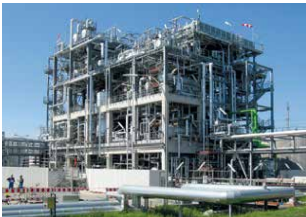
Fig. 1: Propane deasphalting plant (PDA), H&R Ölwerke Schindler GmbH, Hamburg, Germany
