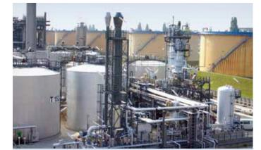
BITUROX<sup>®</sup> PLANT OMV Biturox<sup>®</sup> plant for production of special road paving bitumen
