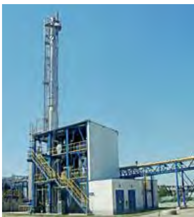
Formalin plant, Dynea Erkner GmbH, Germany, 2015
