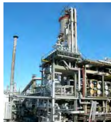
Modernization of crude oil distillation plant RD4, OMV AG, Austria, 2014
