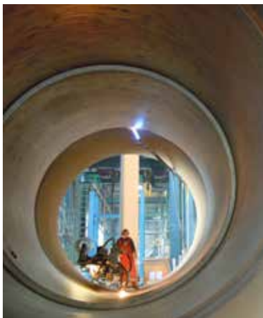
Manufacturing of the new HDS3 reactor at MAN for OMV, Austria 2015
