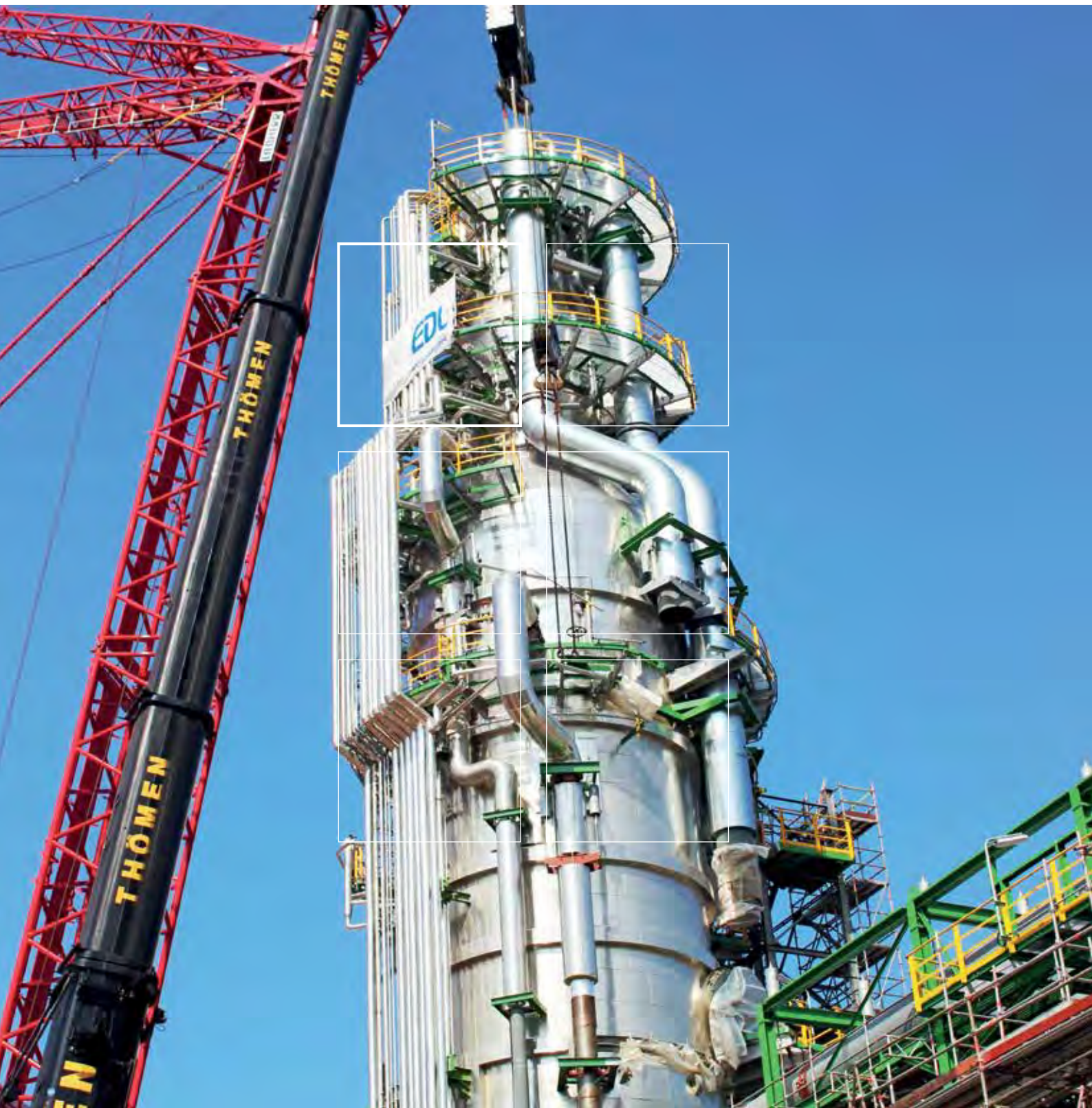
Revamp of the vacuum distillation unit VT3 for PCK Raffinerie GmbH in Schwedt / Germany
