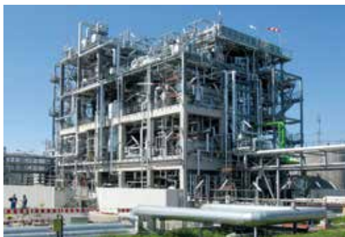
Propane deasphalting plant, H&R Ölwerke Schindler GmbH, Hamburg, Germany, 2011
