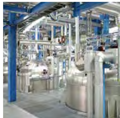
Epoxy resin plant, Leuna Epilox GmbH, Germany
