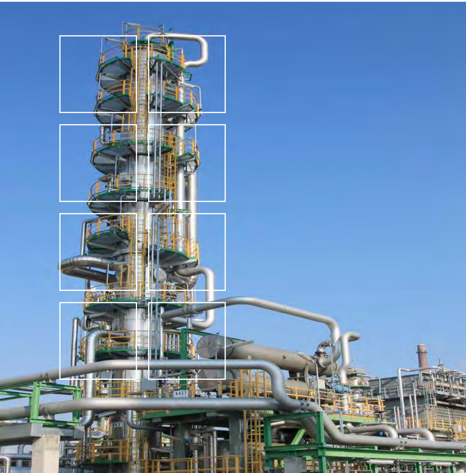
DK2-desulfurization Column, PCK Raffinerie GmbH Schwedt, Germany
