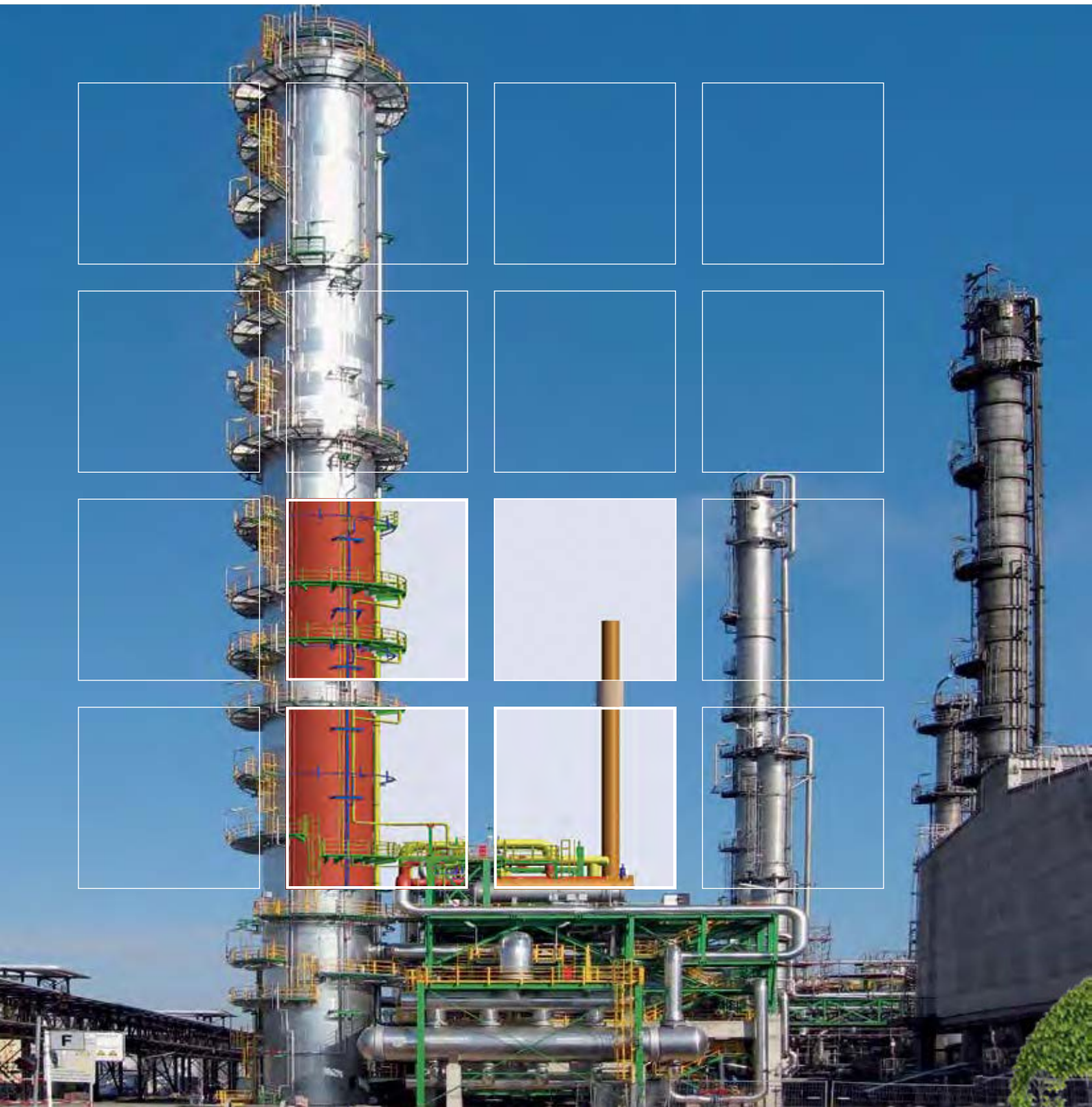
C 3 splitter – with 84 m the highest structure in the region, PCK Raffinerie GmbH Schwedt, Germany
