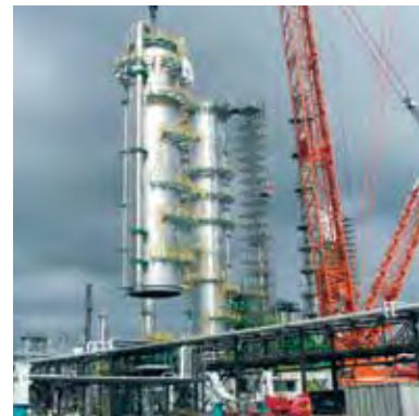
Erection of a two-piece column for PCK Raffinerie GmbH Schwedt, Germany
