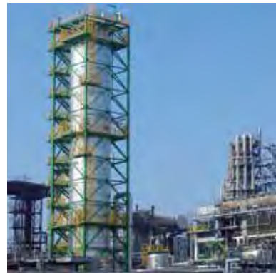
500 m 3 reactor for Desus 1 desulfurization plant, PCK Raffinerie GmbH Schwedt, Germany
