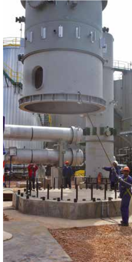
Biturox® plant SAMIR, Morocco, 2011
